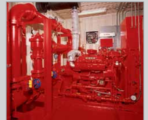
Housed Pre-Pac unit.
