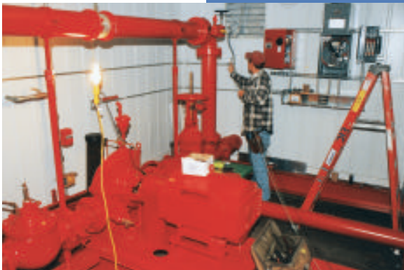
Electrical component installation and wiring.
